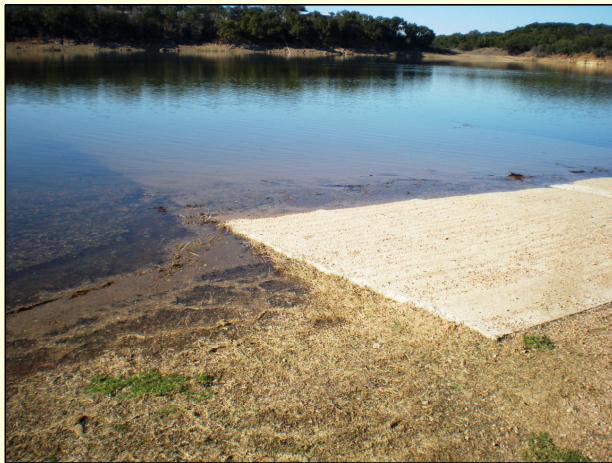
Low-Water Boat Ramp--almost gone.
